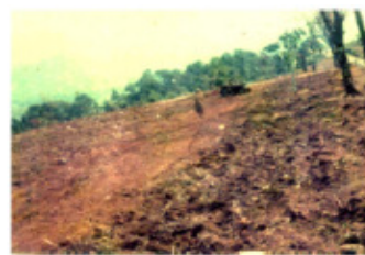
CLEAN PULVERSIED & LEVELLED LAND
